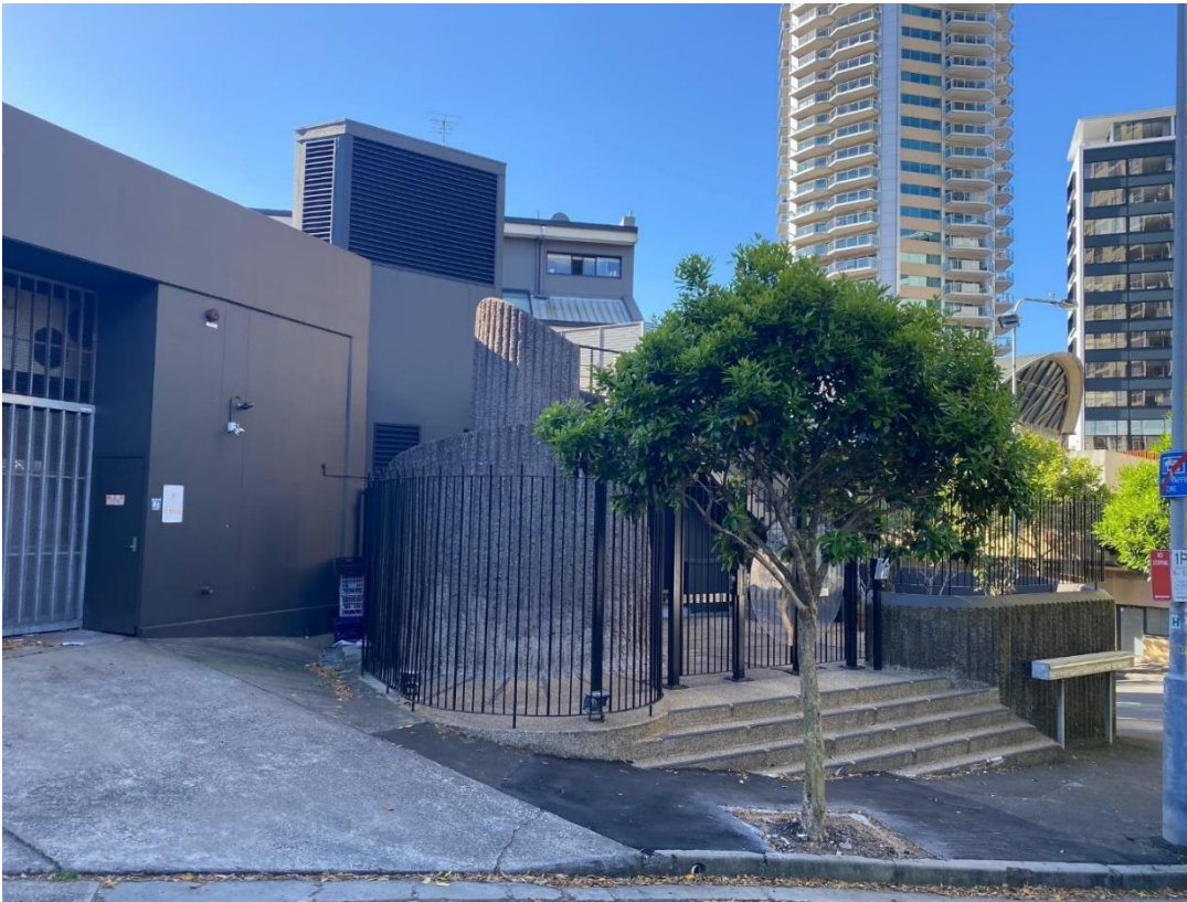
Figure 8. Opposite side of Nimrod St, viewed from site looking north-west
